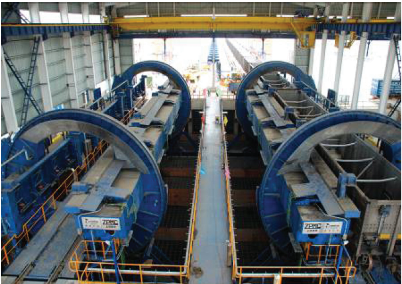
Plate 1. Dual three wagon car dumper unloading facility
